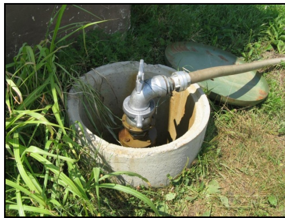
Slika 12: Hidrant namakalnega sistema za priključitev namakalne opreme (terciarnega voda) Figure 12: Hydrant on irrigation system for the connection of irrigation equipment
