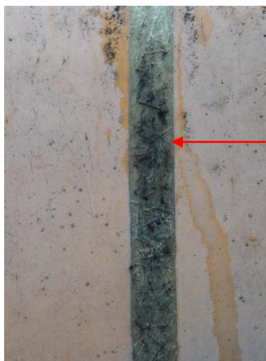
Slika 60: Merilna skala na rezervoarju – skala ni vidna Figure 60: Abscense of fluid measuring scale
