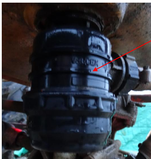
Slika 63: Zastarel, neustrezen izpust, brez zapornega ventila Figure 63: Old, inappropriate release with no valve
