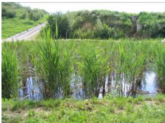
Slika 30: Rastlinska čistilna naprava Dobrava pri Ormožu Figure 30: Constructed wetland Dobrava near Ormož
