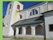
The maternity colony is situated under the projecting roof between wooden beams and this plate, which gives the bats food during the sunny season.
