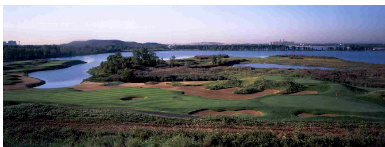
Slike 24, 25, 26: Harborside pred in po sanaciji (Harborside International, 2008)
