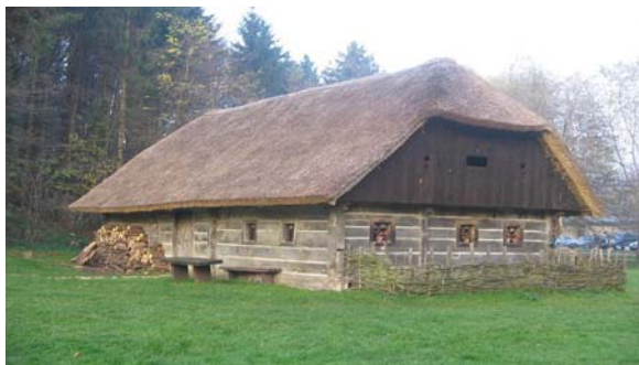
Slika 3: Slamnato ostrešje (Grobovšek, 2009)
