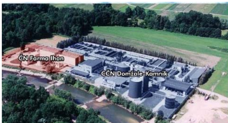
Figure 1- Aerial picture of the Domžale-Kamnik WWTP (CČN, 2007)
