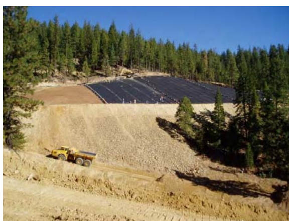
Slika 10: Polaganje vrhnjih plasti (Altoona mine ..., 2009)
