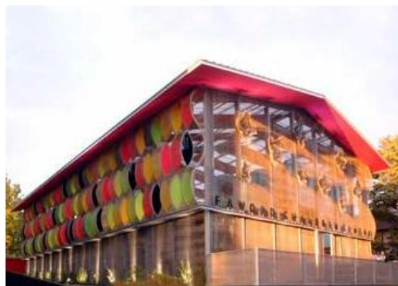
Slika 14: Fawood Children's center (Arcspace, 2016)
