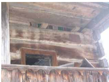
Slika 42: Strop, (a) tram na katerega so s spodnje strani pribite deske, (b) stropni tram in stropne deske
