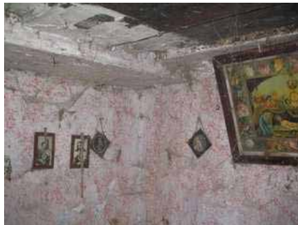
Slika 42: Strop, (a) tram na katerega so s spodnje strani pribite deske, (b) stropni tram in stropne deske
